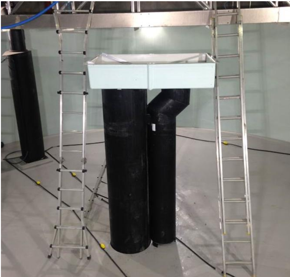
Figure 6. Large drain structures used to rapidly remove dead or moribund fish from the tank center provide a huge benefit to the tank operator but also impact culture volume hydraulics.
