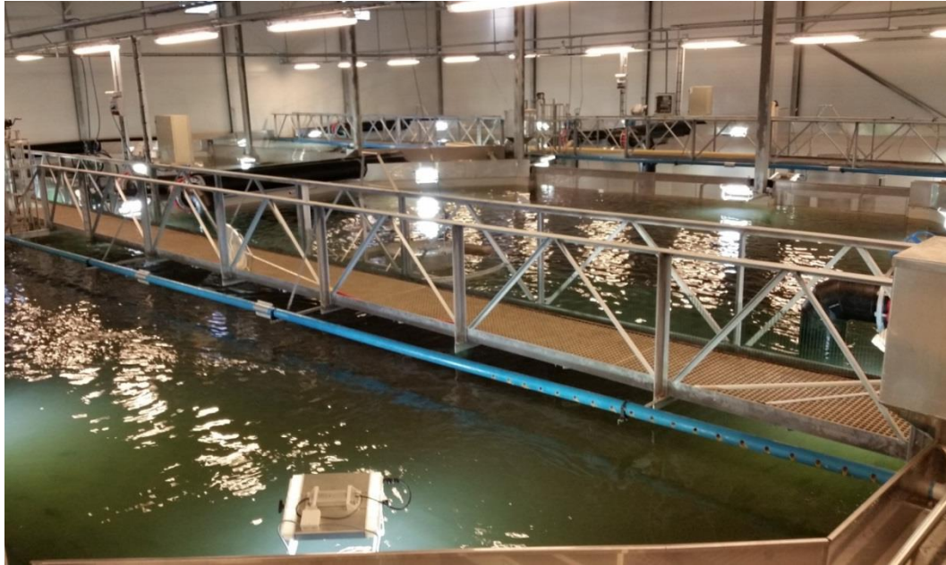
Figure 1. Example of octagonal tanks (14.5 m wide x ~4 m deep) grouped together in one of the recirculating systems at the Marine Harvest Steinsvik hatchery.
