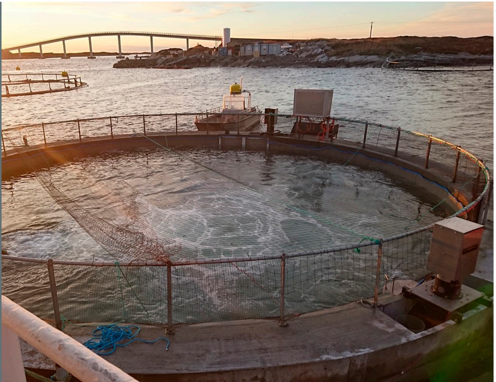
Pilot cage of 1.000 m 3 floating semi-closed concrete sea cage at Gullklakken. Photo © Nekton
