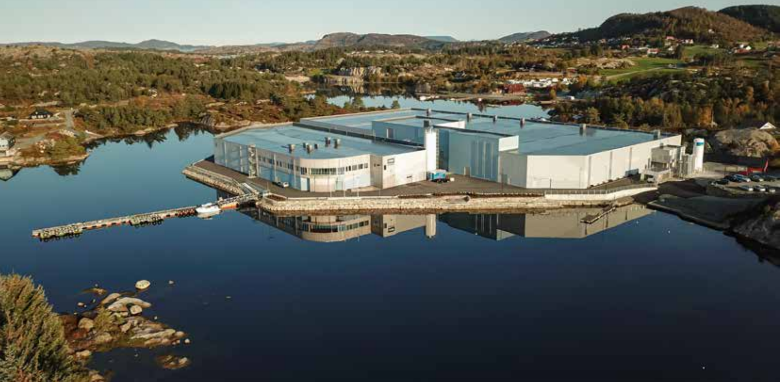
Lerøy Seafoods facility at Kjærrelva, Norway. Photo: ©Lerøy Seafood Group ASA.
