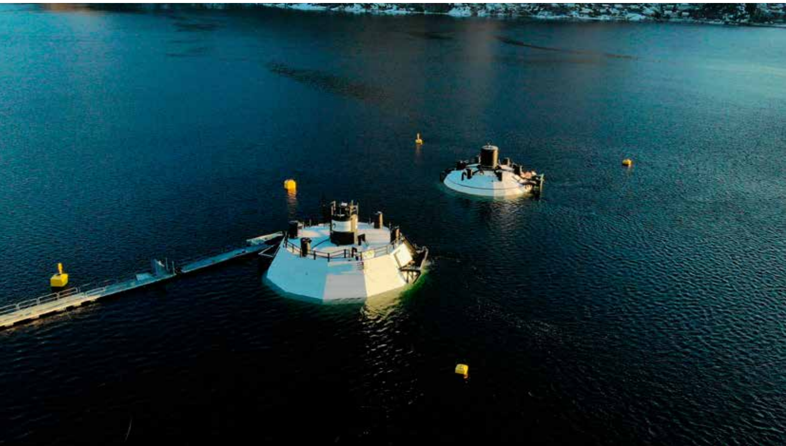
FishGLOBE producing post-smolts in their uniquely designed closed-containment aquaculture systems in Lysefjorden. In the picture, the 2021 system can be seen to closest to the left, while the 2019 system is to the right. Photo: Meyer Media, ©FishGLOBE.
